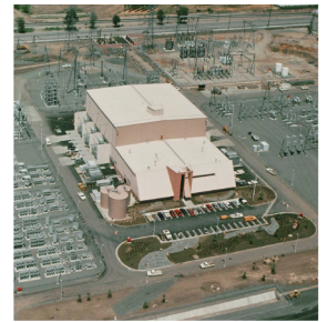
Typical AC/DC Converter Station
