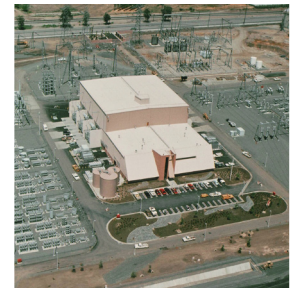
Typical AC/DC Converter Station
